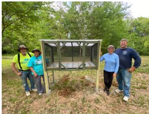
The butterfly habitat is installed and operating nicely in Jackson County Park. Pictured (L-R) Builder John Horning, with wife, Gail; project planner Wilma Brockett, and helper Dan Schults. Photographer: Wilma Brockett.
